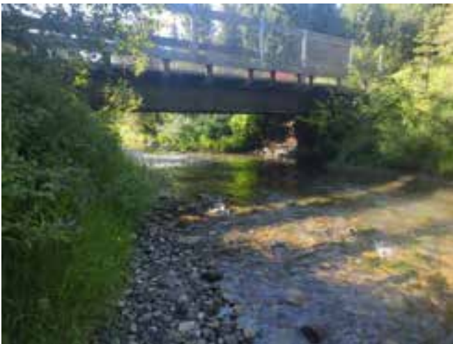
Photo 1: View of the bridge over Lizard Creek. July 28, 2022
